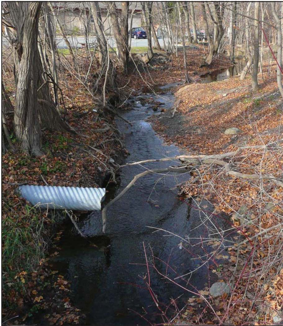
A Drainage Pipe Feeding into Witch's Brook before It Empties into the Wawayanda
