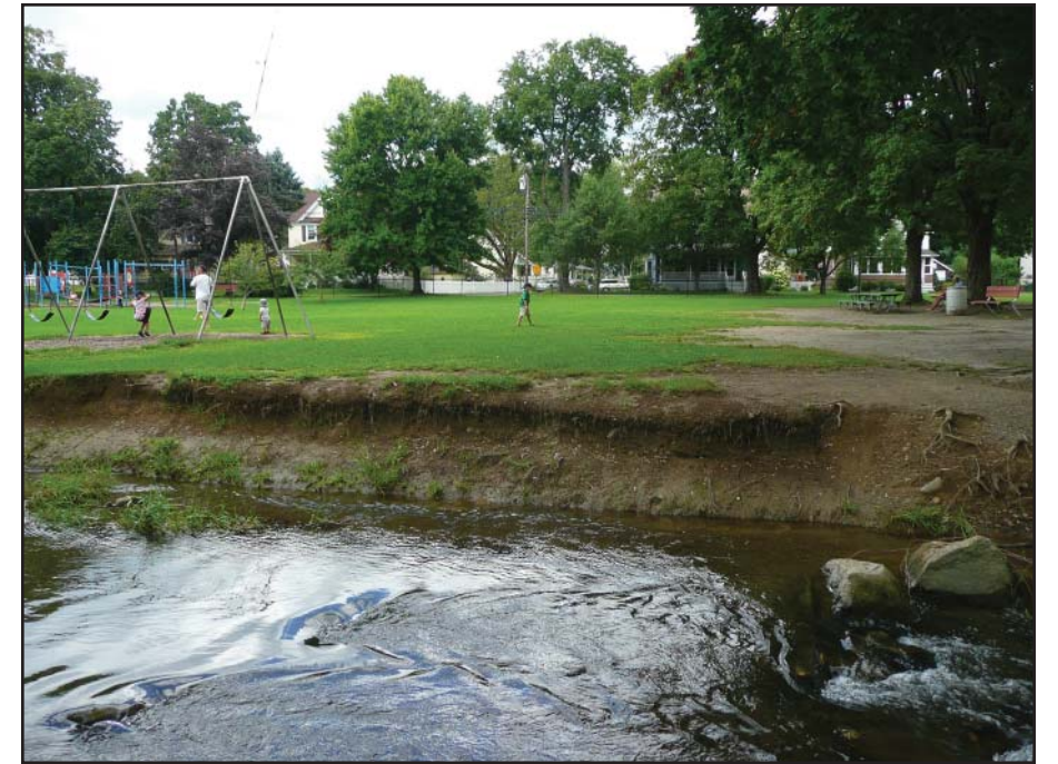
Severely Eroded Banks of the Mistucky Creek in Stanley Deming Park
