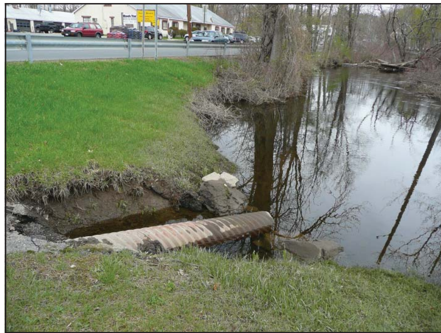
An Eroded Ditchline and Pipe Outfall into the Wawayanda Creek at Memorial Park Lake
